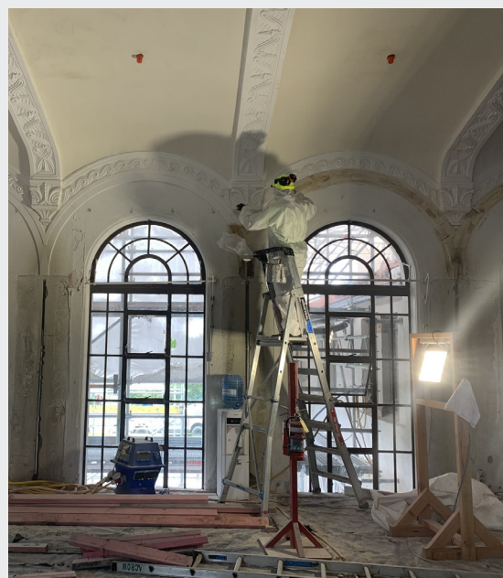
Experts repair the original plaster motifs in the Refectory.
